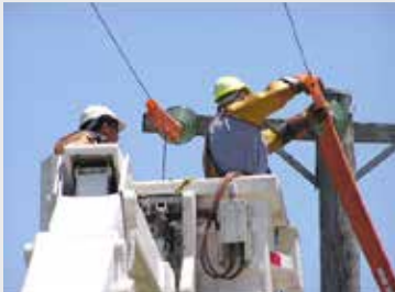
Live line work (elevated electric fields also)
